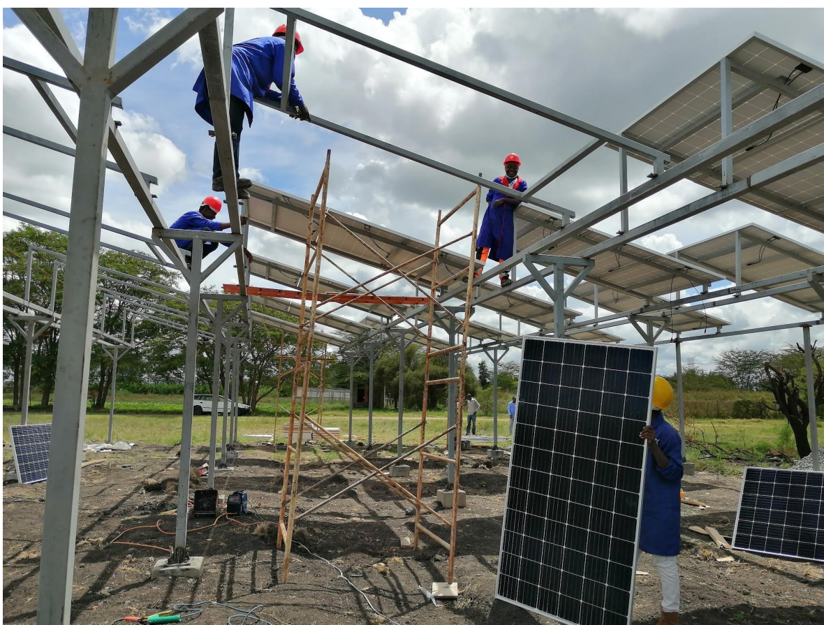
The Chloride Exide team installs solar panels 3m above the ground on custom-designed scaffolding at Latia Farms, Insinya, Kenya. Photo: C. Lamanna (ICRAF).
